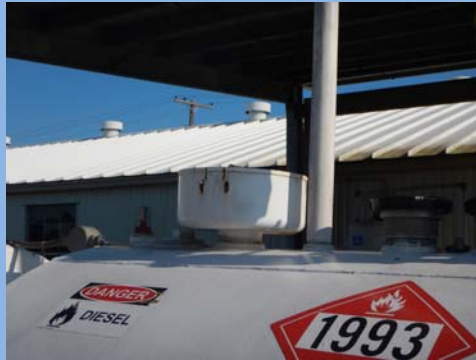
Damaged fill drip pan needing repair
