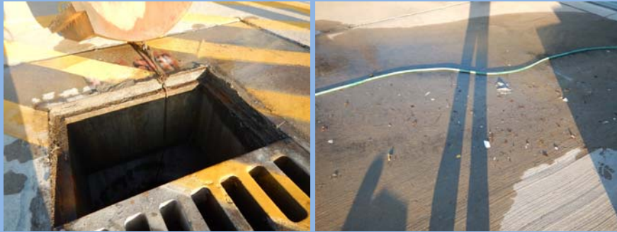
Debris in the wash rack area and drain.
