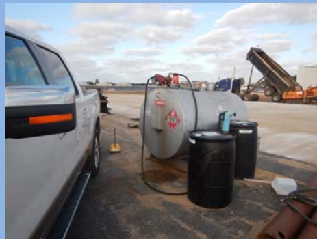
Leak from fuel nozzle.
