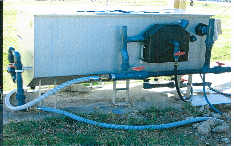
Pretreatment unit has been connected inline.
