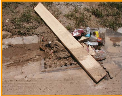
BAD BMP: Debris covers a storm drain interfering with drainage. Dirt is also being allowed in our waterways. This is what we do NOT want to find when we are out on job-site inspections.
