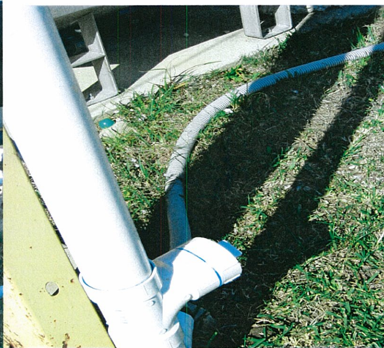
Pretreatment unit has been connected inline.
