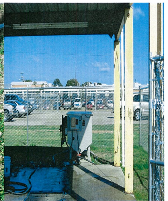
Pretreatment unit has been connected inline.
