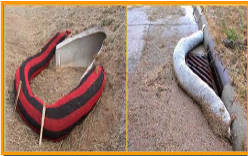
GOOD BMP: These wattles protect the storm drains. This is what we expect to find when we are out on job-site inspections.
