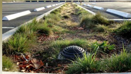
Picture from the following web site http://www.sonomacity.org/Services/Q-Z/Stormwater-Maintenance/Stormwater-Program-Post_Construction-Landing-Page.aspx
