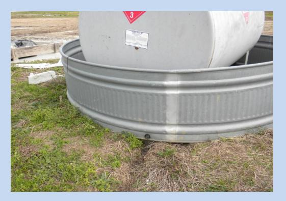
The drain port is left open. It must remain closed to prevent discharge of oil.
