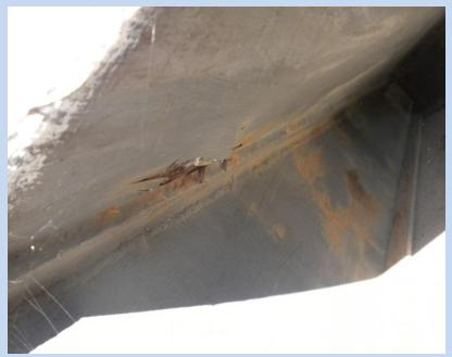
Nicely Painted bulk container has corrosion at base that needs to be addressed.
