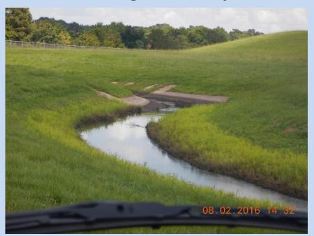
Staining on banks of ditch is evidence of release. Need to notify Environmental Compliance or Security.
