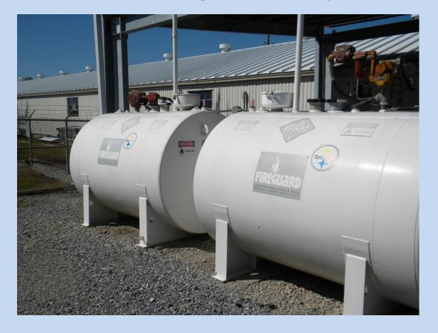
Double-walled containers have faded labels.
